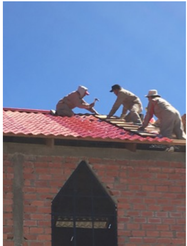
A NEW ROOF FOR NUEVA JERUSALEM VIACHA
